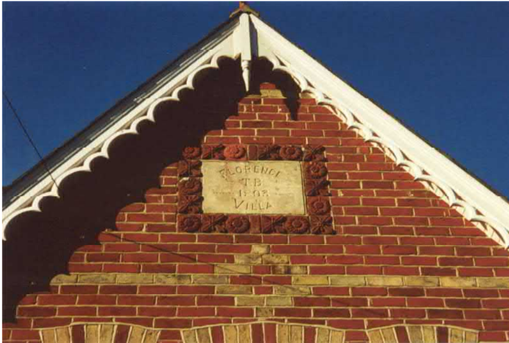
Figure 2: A local house built with Rowland's Castle multi-coloured bricks and terracotta circa 1893
