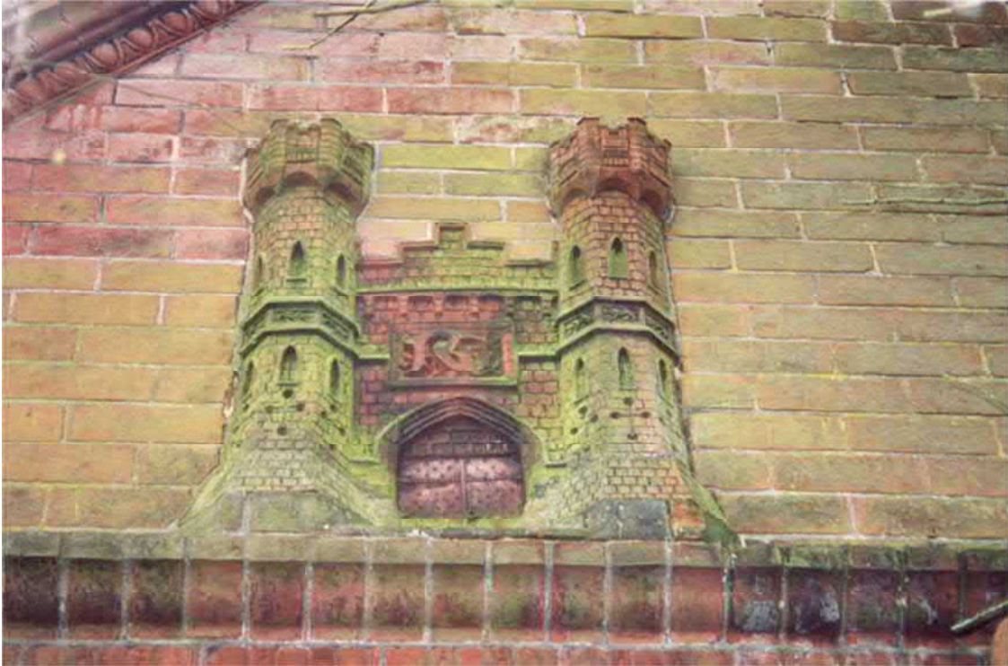
Figure 11: Elaborate terracotta work on the east gable wall
