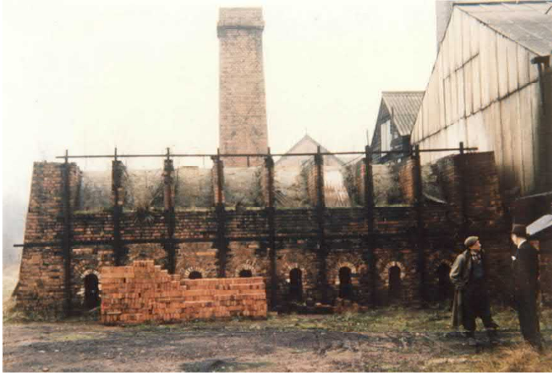
Figure 10: Photograph of the Hoffmann kiln at Rowland's Castle (1969)
