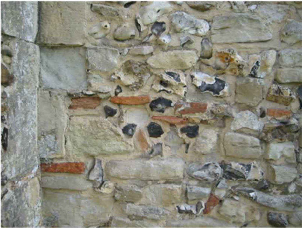
Figure 1; Reused Roman bricks in the wall of Warblington Church
