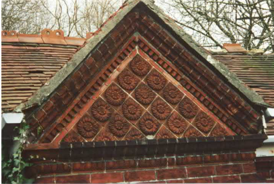
Figure 6: The office built in the late nineteenth century showing the highly decorated pediment above the porch
