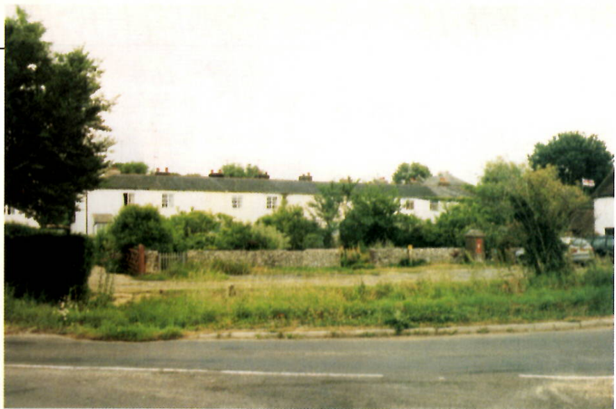
Once known as 'The Barracks', John Cannings' row of foundry workers cottages at Dean Lane End still have the pretty iron window frames which were cast at Finchdean Ironworks.
