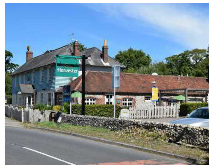
The Harvester public house was originally a private dwelling, and has had several extensions. The single-storey flint extension with a clay tile roof is an appropriate vernacular aesthetic. The low flint wall is an attractive frontage to Whichers Gate Road.
