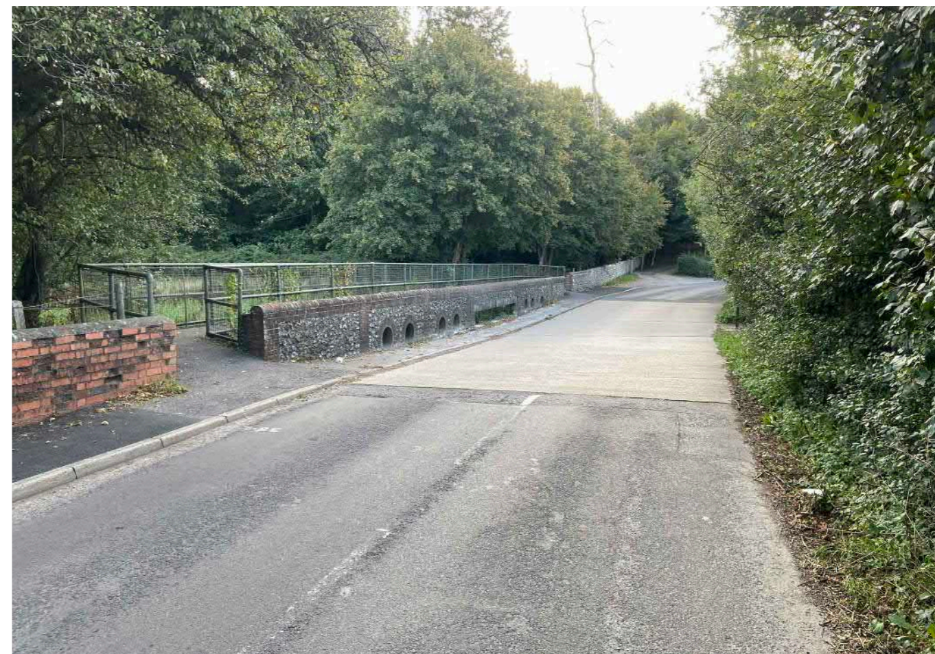
Where the Lavant stream crosses Woodberry Lane traffic movement can be impeded after storm surges
