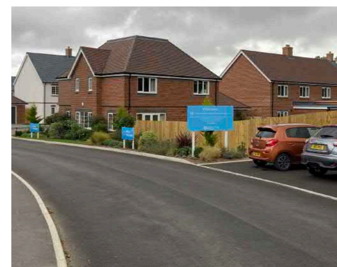
Close-board fencing, standard concrete road kerbs and a dominance of parked cars can detract from the streetscene
