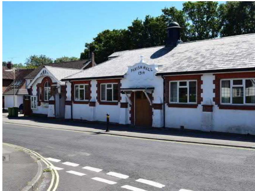
The Parish Hall is a well-used community venue, located on Links Lane, and not visible from The Green.
