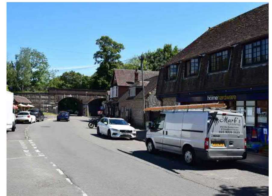
The eastern end of the 'Historic core' terminates with the double arches of the railway bridge. The village general store, hardware shop and cafe are also seen in this view.
