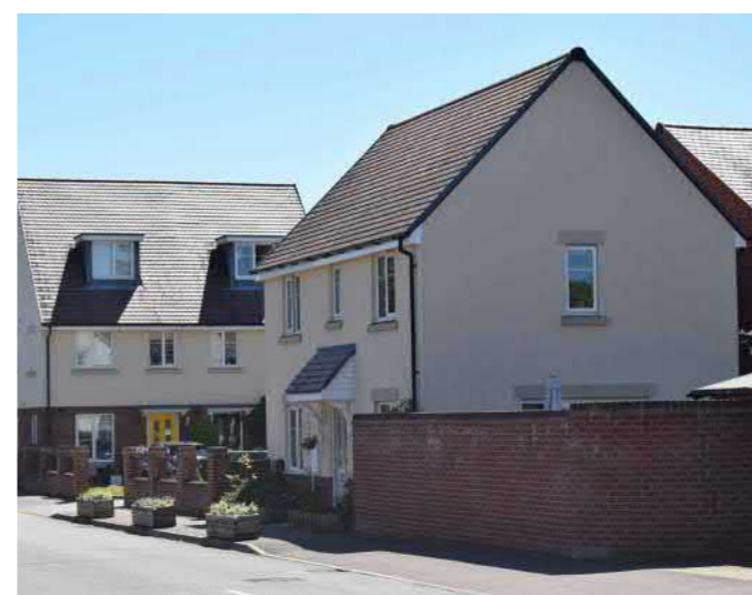
Blank walling of rear gardens siding onto the public realm at Oaklands Avenue.
