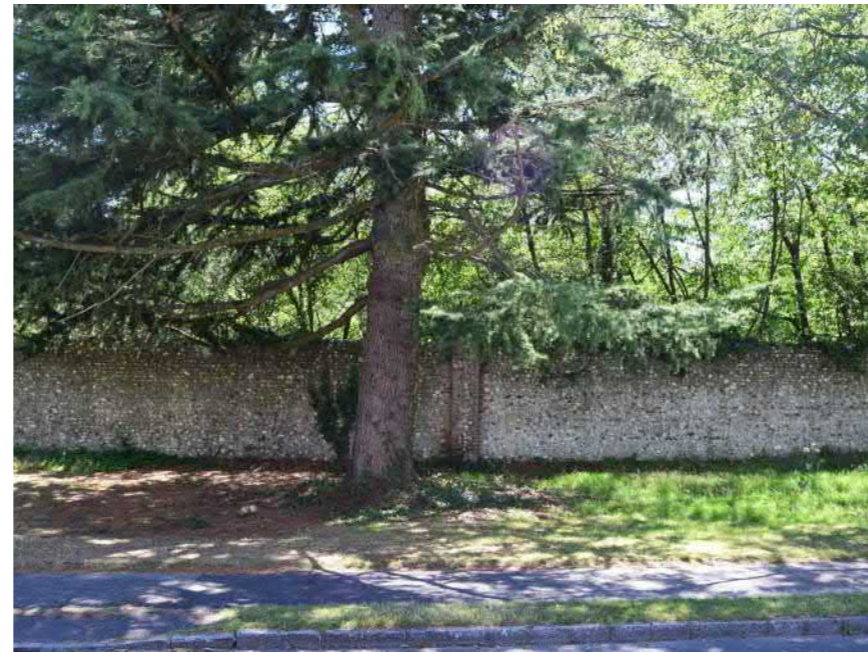
The notable flint boundary wall to Deerleap, running almost the whole length of the village green, along its southern side
