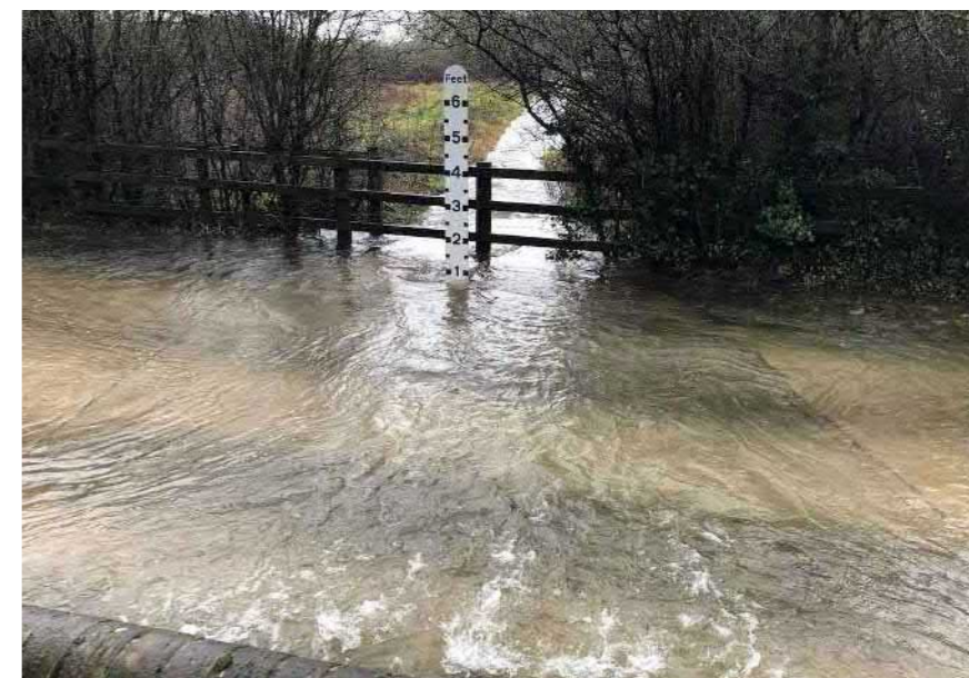
Flood waters surging across Woodberry Lane
