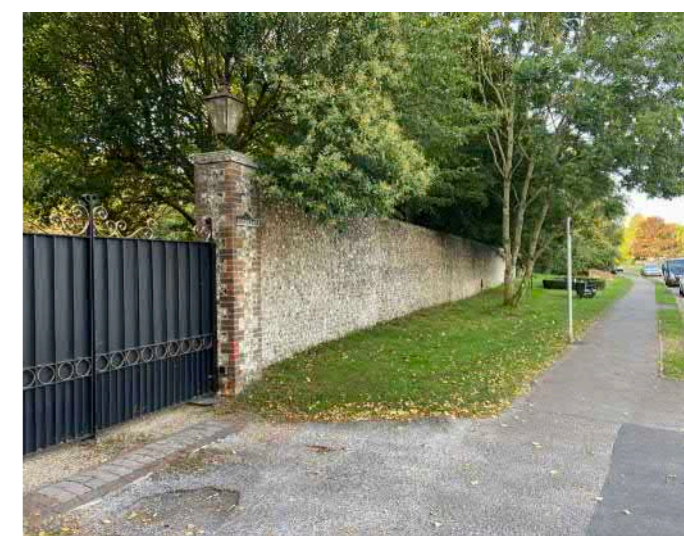
Flint is a characteristic building material, most notably the tall boundary wall of 'Deerleap'
