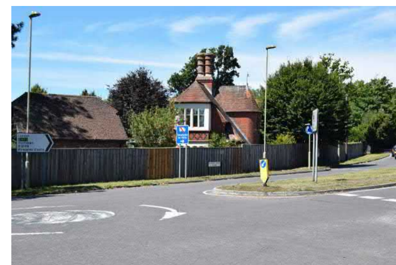
The setting of some attractive housing is much compromised by highway infrastructure
