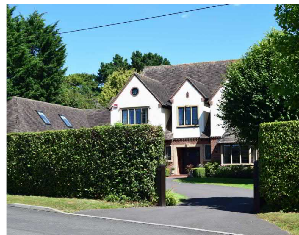
Development should aim for interesting roofscape, but avoid overlooking dormer windows and rooflights
