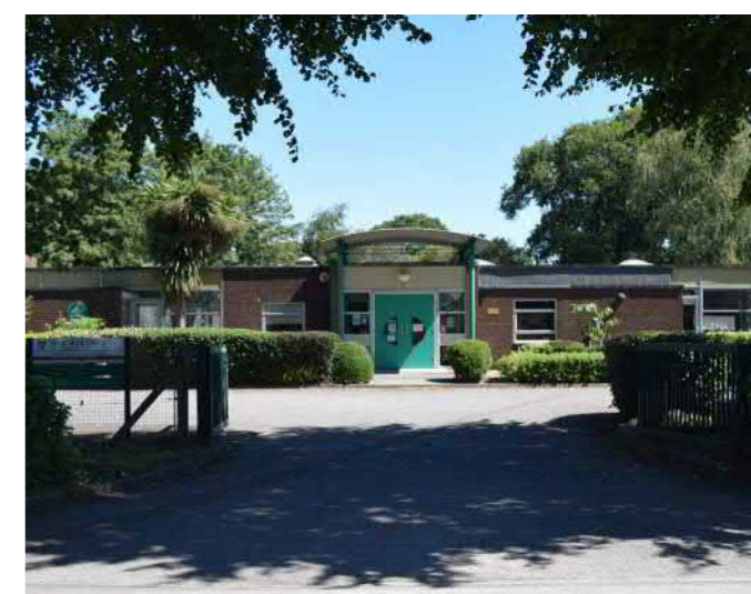
The primary school is a low-level building with a large footprint, set in extensive school grounds, partly asphalt surfaced alongside a playing field surrounded by mature trees.
